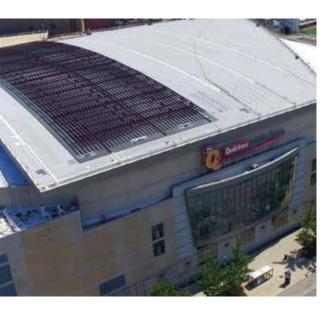
The 24 year old 170,000 square foot original roof of Quicken Loans Arena in Cleveland, Ohio-better known as "The Q"-received a new lease on life thanks to a roof restoration by Beachwood, Ohio-based Tremco Roofing and Building Maintenance and contractor Warren Roofing of Walton Hills, Ohio. The two phase project, completed in the summer of 2017, effectively doubled the service life of the roof with Tremco Roofing's liquid-applied AlphaGuard® MT roof restoration system.
