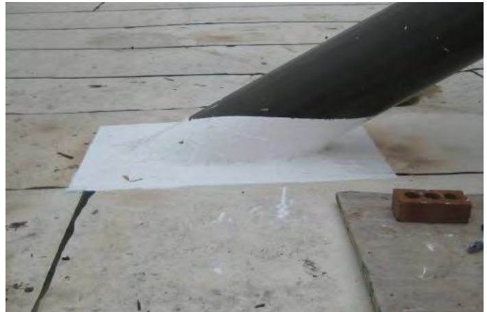
Penetrations on MB roof systems can be flashed with AlphaGuard as well.
