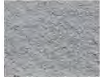
CSP 3 (Light Shot blasting)
