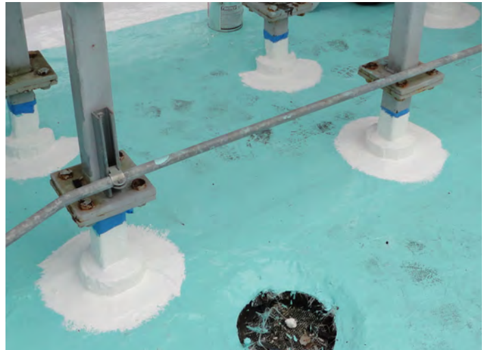
Flashing pipes and stands are easy and seamless.
