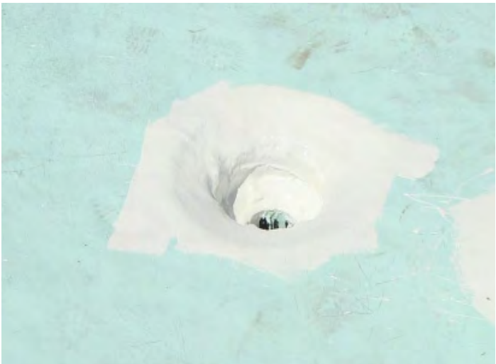
For concrete and insulated systems, extend AlphaGuard into the drain bowl. Ensure that the drain bowl is prepared per requirements.
