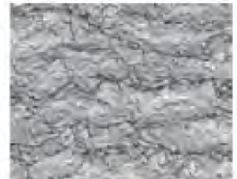
CSP 9 (Heavy Scarification)
