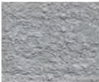
CSP 4 (Light Scarification)
